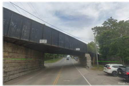
West Ave. at Atwater Park. Trestle clearance: 10'-6" east bound, 12'-3" west bound.
